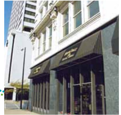
Main Street Coffee House was awarded a Façade and Streetscape Improvement Grant for new awnings.
